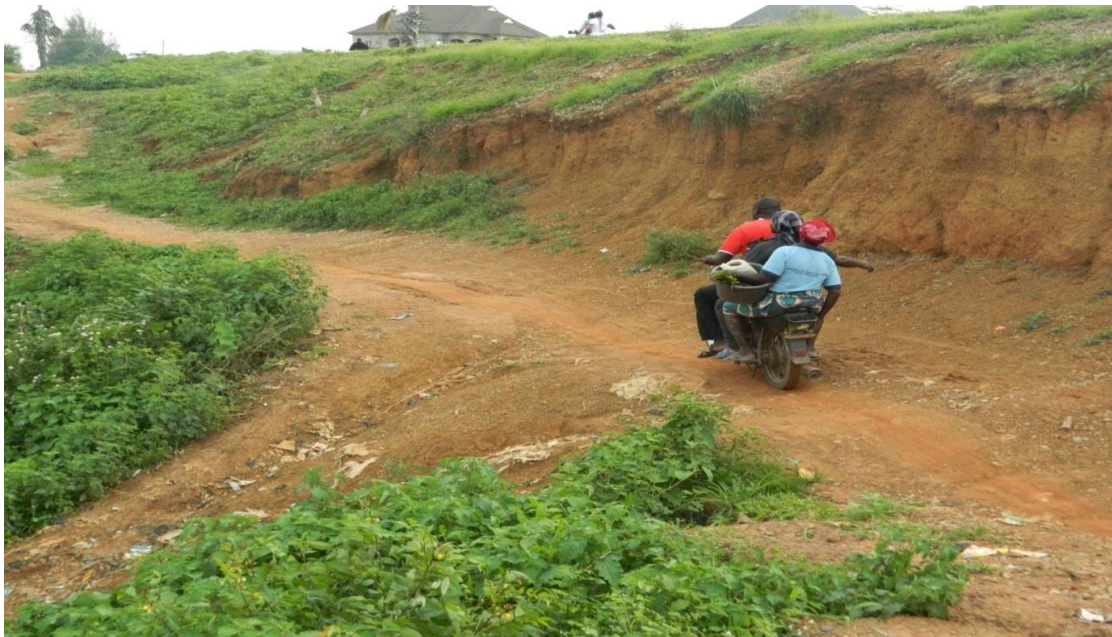
Figure 6: Pictorial View of Gully Affected Area of Goni-Gora before the Rail.
