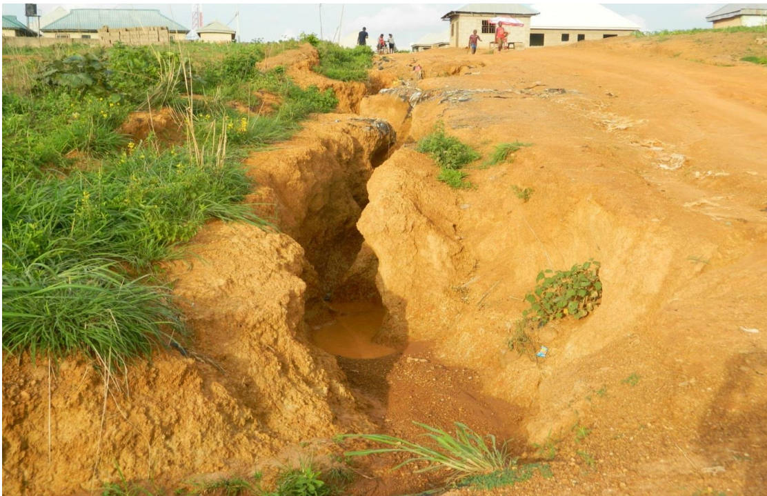
Figure 7: Pictorial View of Some Gully Erosion Sites in Chukun.
