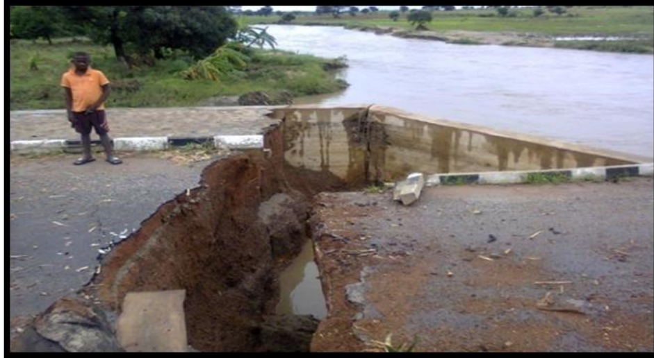
Plate 12: Bridge linking other Villages. Source: (Buba Y. Alfred 2012)
