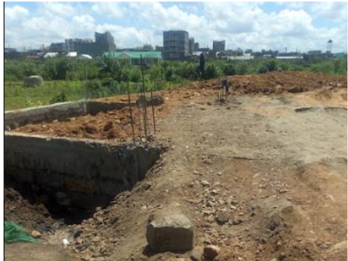
They have already started laying the foundation for their facility.
